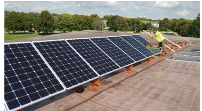
Photo: Installing solar panels at the Warner Park Community Recreation Center
